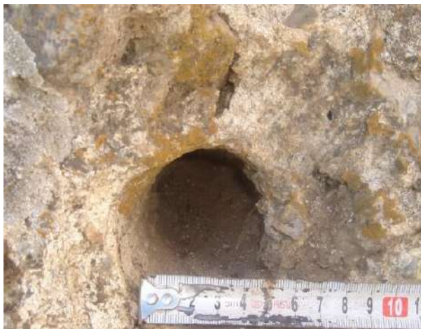
Fig.12: Perforation view of the scaffolding construction.
