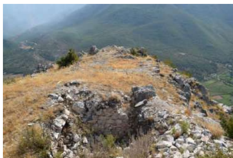
Fig. 33a-General view of Scanderbeg's water tanker and Tower;
