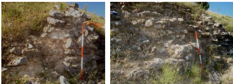
Fig.10-11: The external wall I and II of the tower-tract C.
