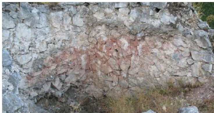
Fig. 27. View of the water tanker
