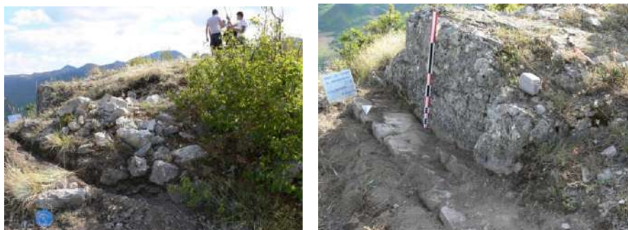
Fig. 34a-b-View of the northern and eastern wall of Scanderbeg's tower
