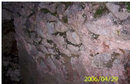
Fig. 23. View of the water tanker of Modrica
