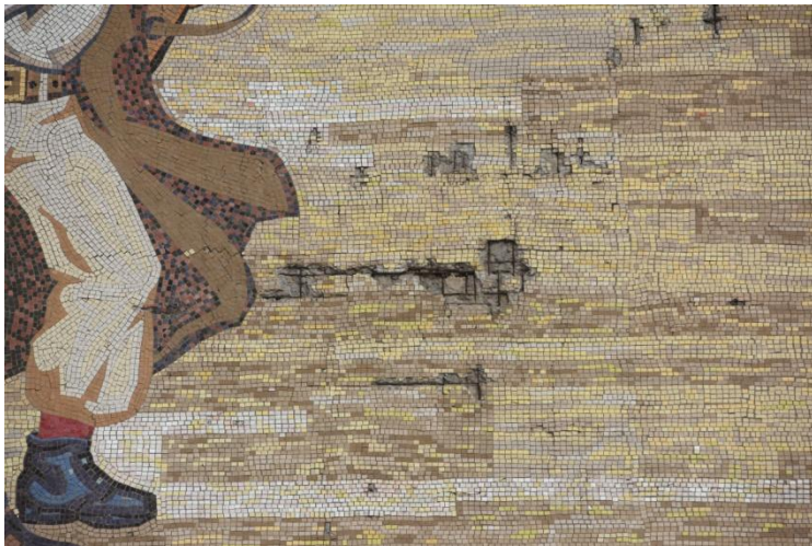
Fig. 5. Photograph of tiles missing from the mosaic on the National Historical Museum, Tirana. Photo by Alban Hajdinaj. Image courtesy of the artist.
